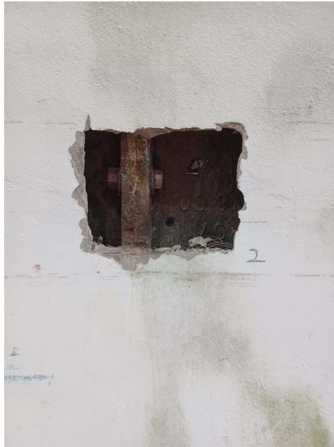
Plate 5: General view of exposed tunnel lining. Test Location 2
