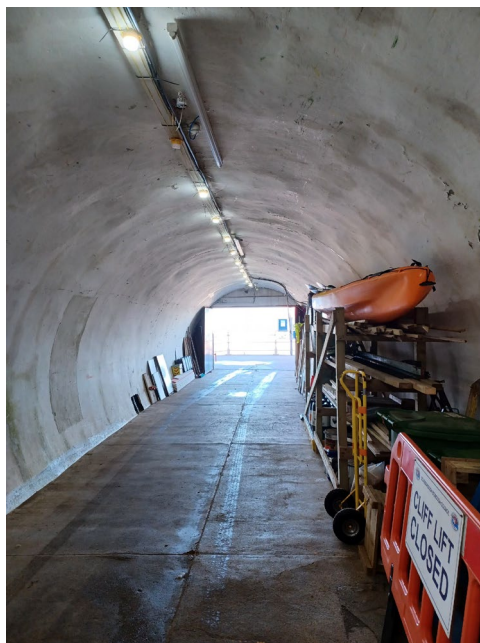
Plate4: General view of tunnel-towards the beach
