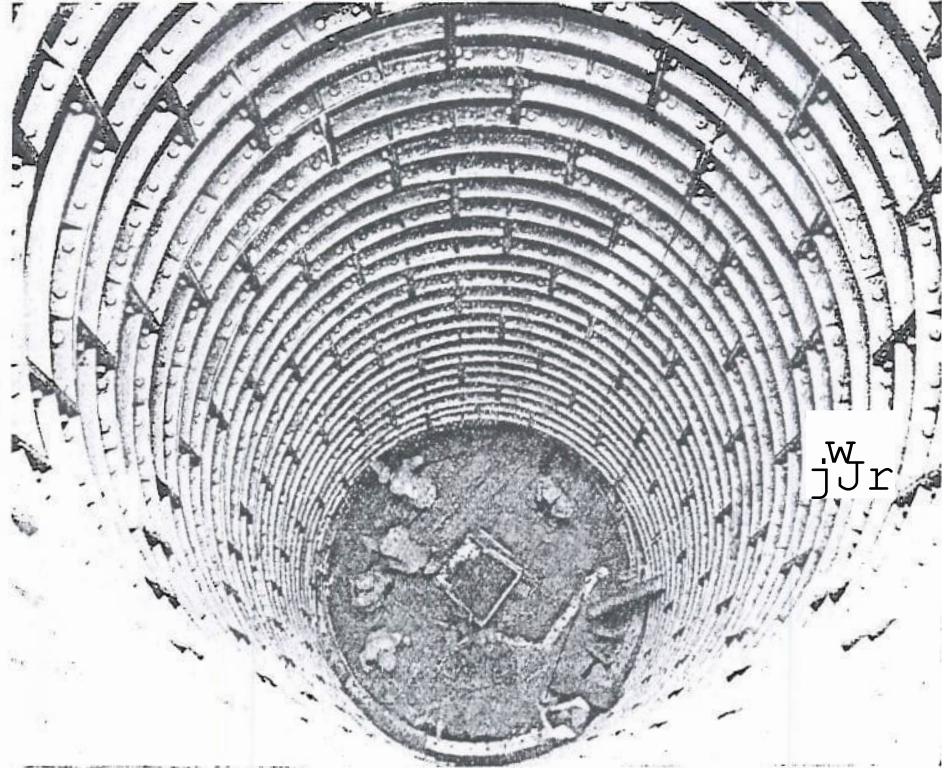
L 4 Northern Echo **photograph. LOOKING DOWN SHAFT, 59 FT. DEEP.
