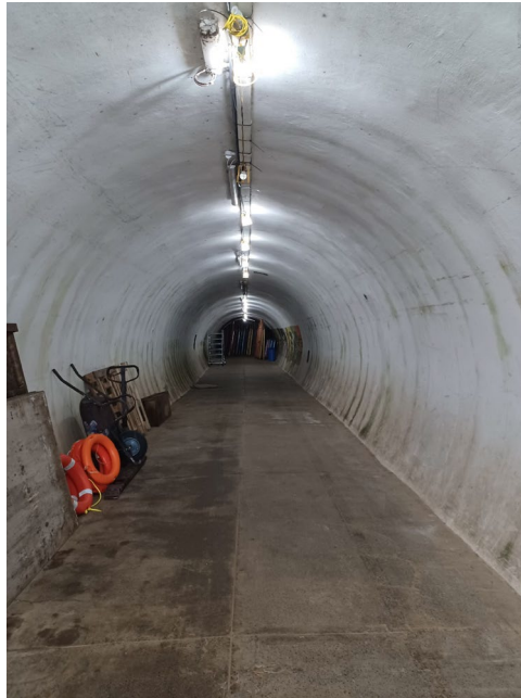
Plate 3: General view of tunnel-towards the lift shaft base
