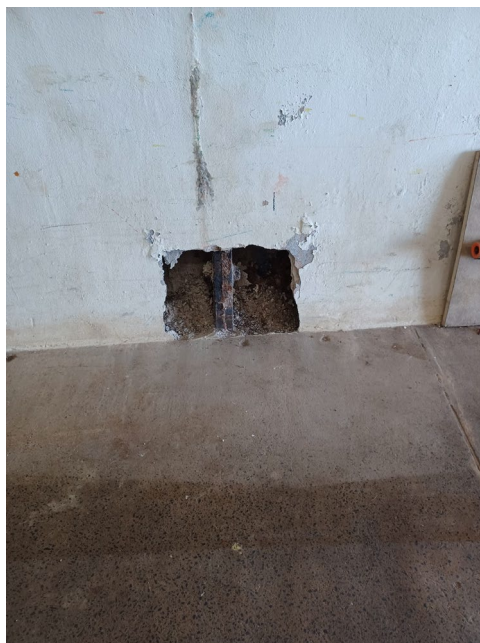
Plate 6: General view of exposed tunnel lining. Test Location 1
